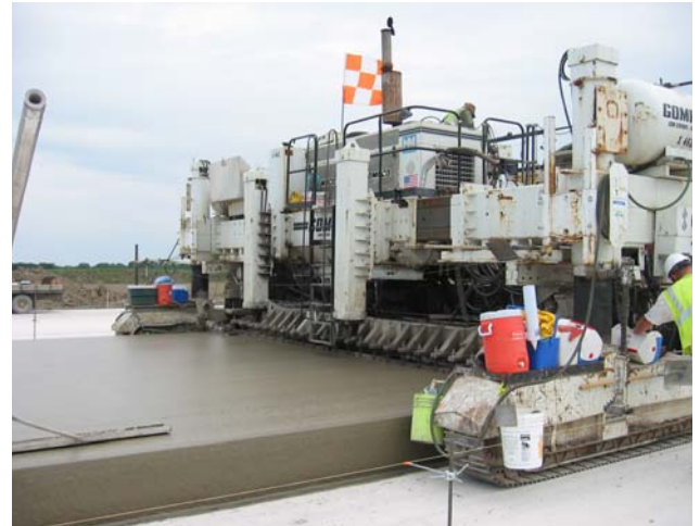
Smooth Paving on a Stable Platform
