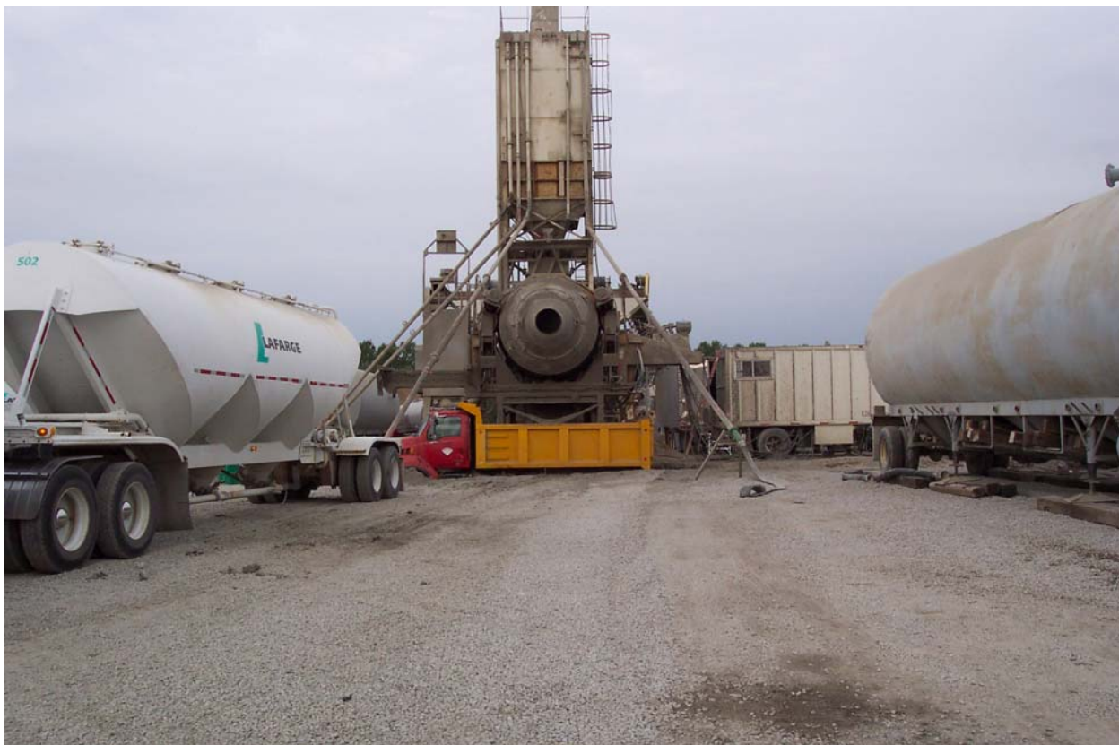
Double Drum Batch Plant
