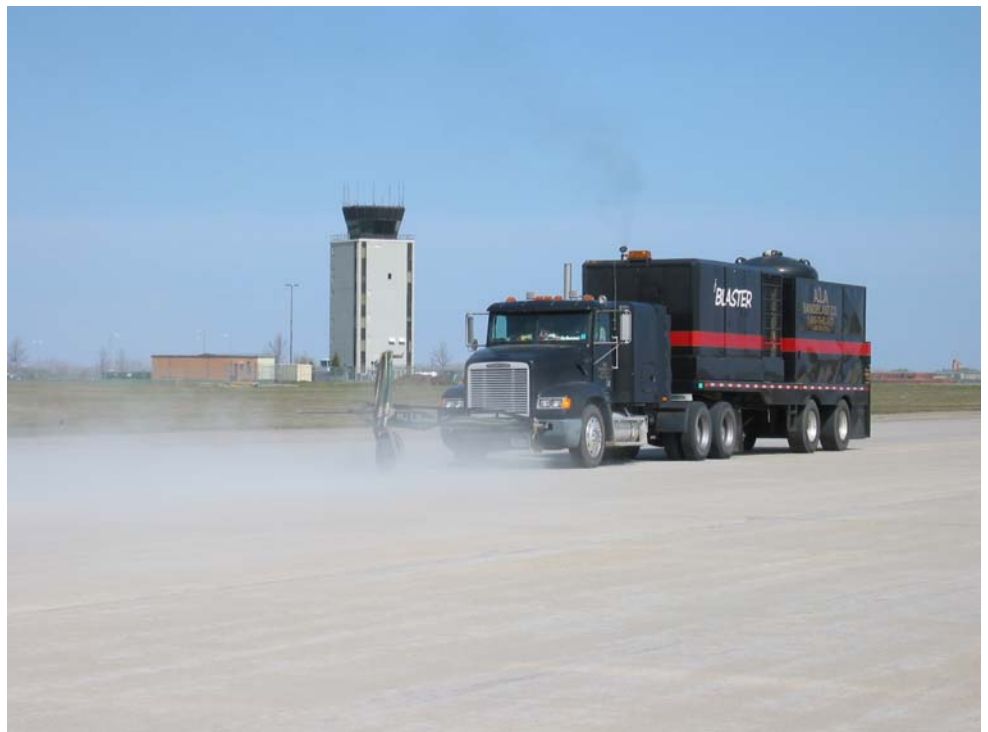
Sandblaster Removing Taxiway Markings for Conversion to a Temporary Runway
