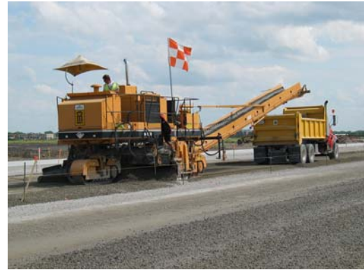
Trimming Aggregate Subbase
