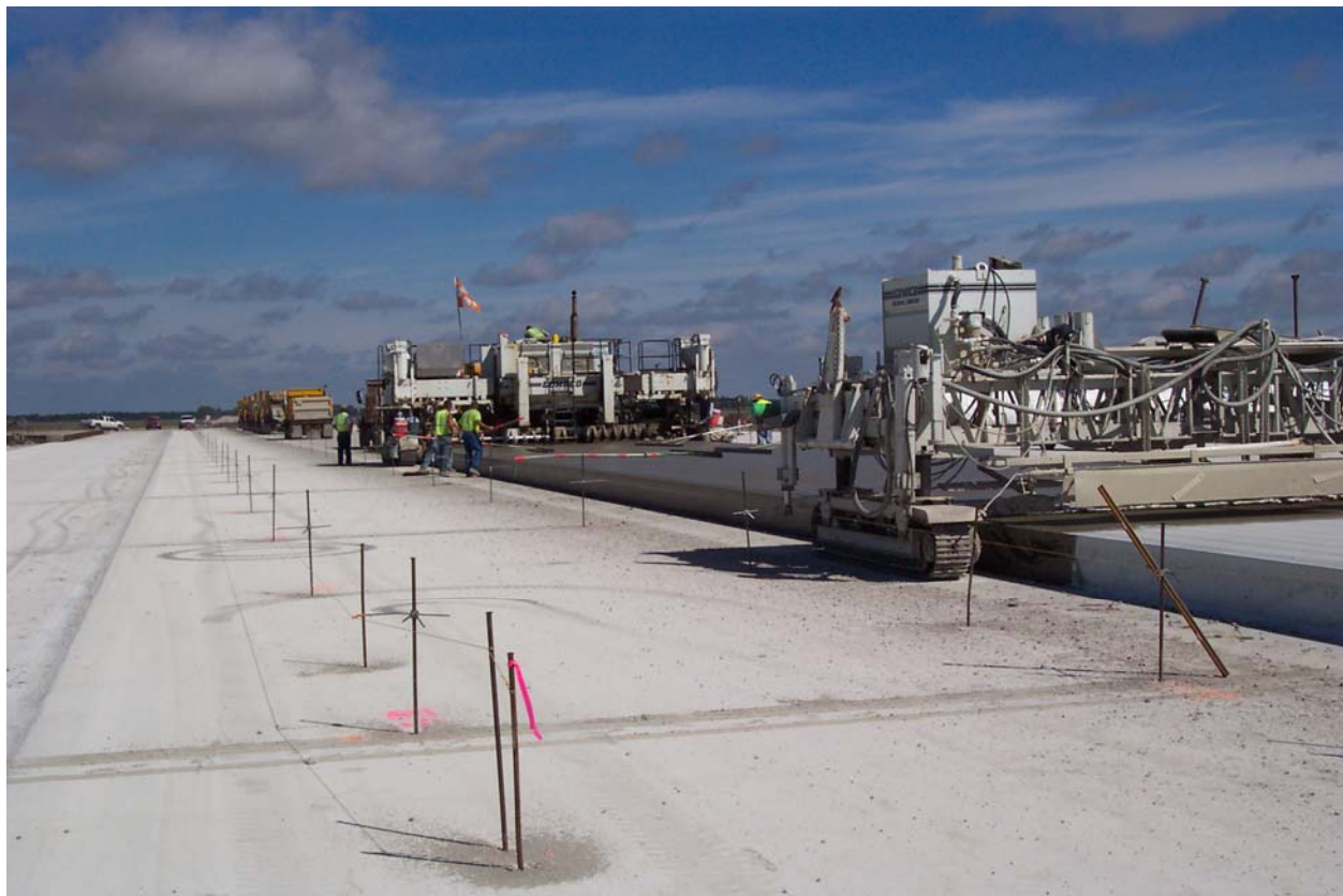
Smooth Paving with Consistent Concrete that was Compatible with Shafer's Equipment
