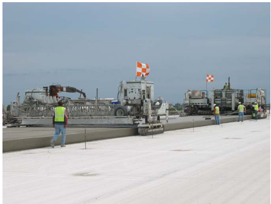
Smooth Paving with Well-Graded Aggregate Mix
