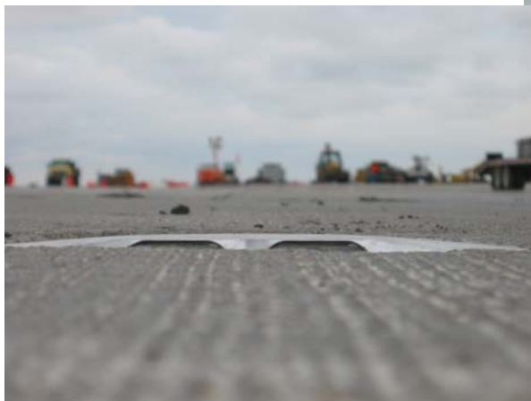
Perfect In-Pavement Light Installation
