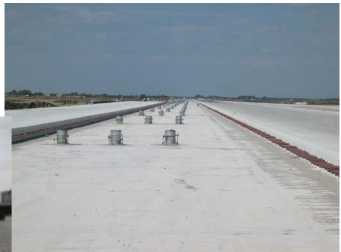
Touchdown Zone Light Bases Ready for Paving
