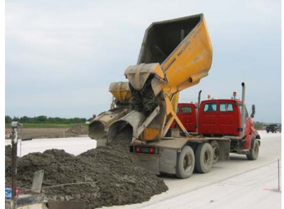
Agitor Trucks Placing Concrete
