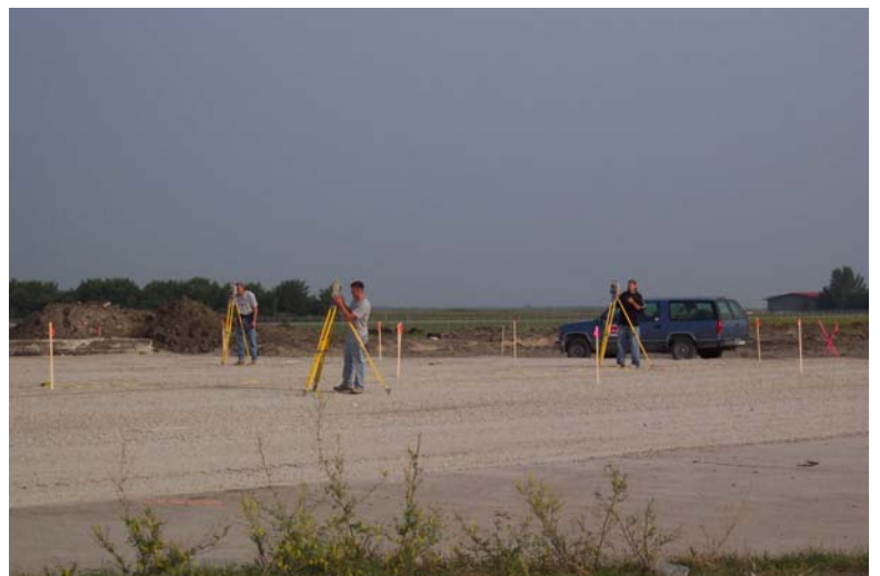
Ulteig Survey Crews Setting Stringline Hubs
