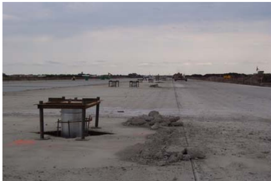
In-Pavement Light Bases Held Securely with Alignment Jigs
