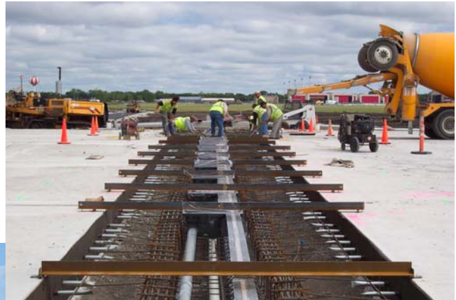
Placing Concrete for the South Arresting Barrier
